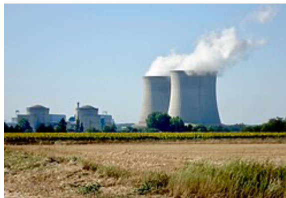
France's Saint-Laurent nuclear facilities, with two 900 MW civilian nuclear power reactors, on the left, and their cooling towers on the right. Source: Saint-Laurent Nuclear Power Plant, Wikimedia , 2022.
