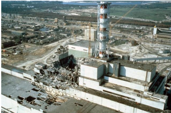
After the explosion: Reactor No. 4 at Chernobyl Nuclear Power Plant. Behind it—intact—is Reactor No. 3
