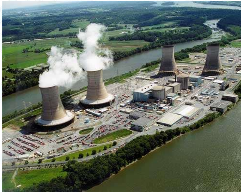
French nuclear electrical generation facility in the Rhone valley
